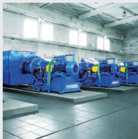
Twelve blowers of DA 340 type that work in Poznań Central Sewage Treatment Plant; pressure rise: 65 kPa installed power: 2400 kW
